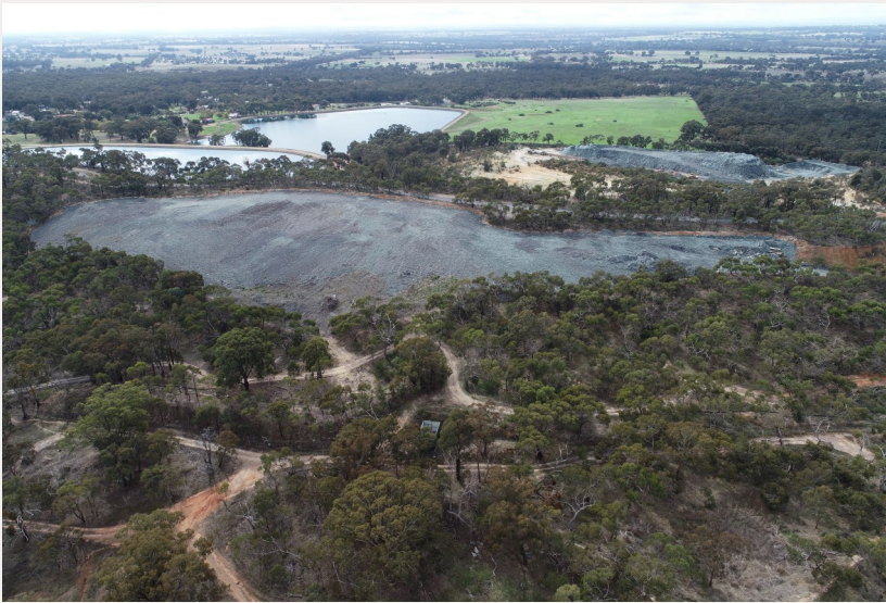
Left: Davis Pit Rehabilitation works— prior to placement of subsoil. Visible is the completed backfilling with inert underground waste rock.
