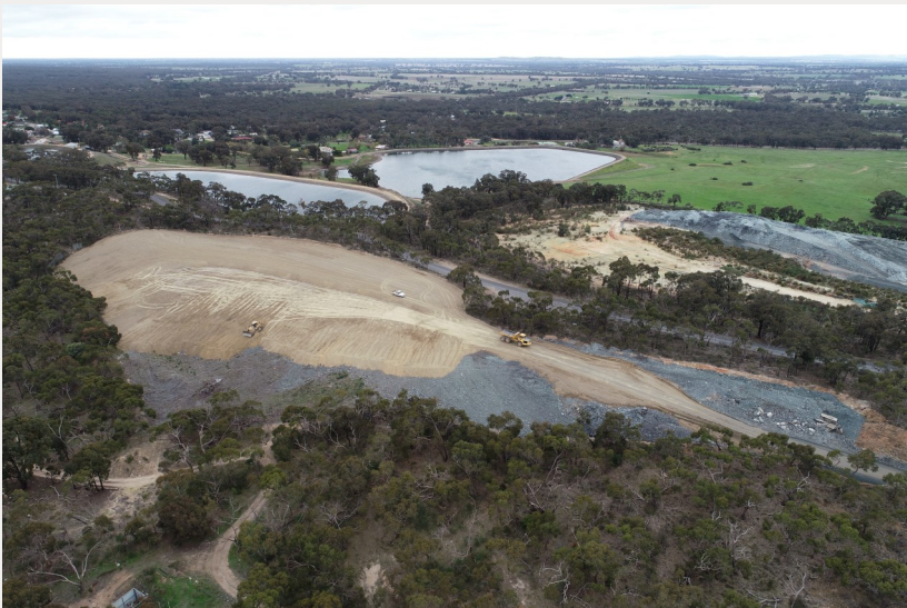
Left: Davis Pit Rehabilitation works during placement of subsoil.
